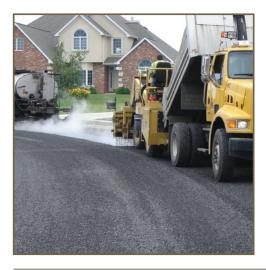
**Description & Scope:** Annual road seal work where select roads are maintained through chip and fog seal treatments. Surface treatments are a two step process where crack seal and patching are completed in phase one and chip seal and fog seal treatments in phase 2.
