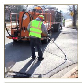
**Description & Scope:** Regular maintenance work of asphalt roads. Work includes identifying cracks, routing, cleaning and filling cracks with tar seal. Scope includes 2017 crack seal roads and 2018 slag seal road preparation.
