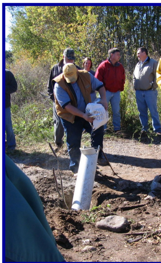
Bentonite chips being poured into a well during abandonment.
